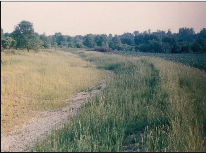
A grassed diversion is planted to redirect water from a slope and also traps nutrients and sediment in runoff
