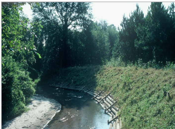
A stream revetment was used to reduce and prevent streambank erosion along with revegetation
