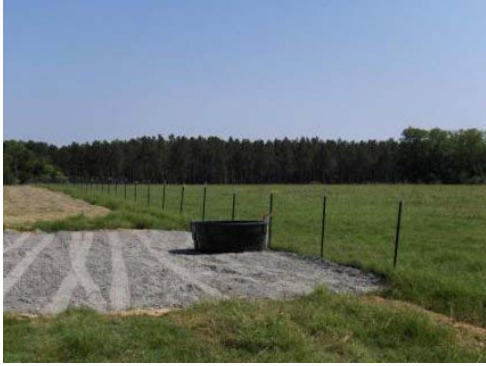
Heavy-use-area limits soil erosion around watering trough
