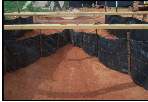
Check Structure Installation over Bare Soil
