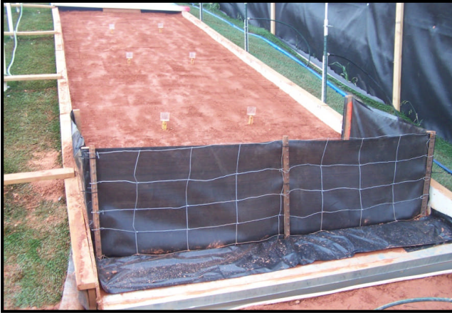
Test Slope Prepared and Fence Installed
