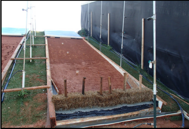
Test Slope Prepared and Straw Bales Installed
