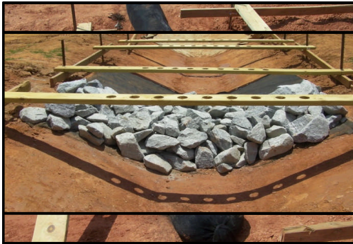
Check Structure Installation over Bare Soil
