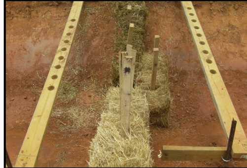
Check Structure Installation over Bare Soil
