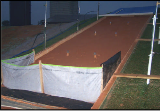
Test Slope Prepared and Fence Installed
