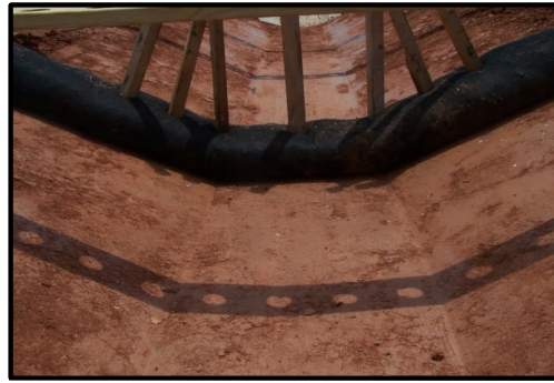
Check Structure Installation over Bare Soil
