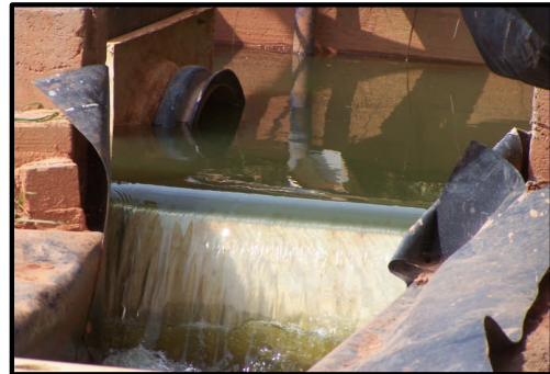
Initial Flow & Inlet Weir
