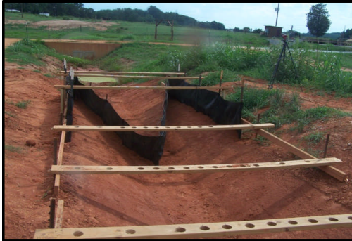
Check Structure Installation over Bare Soil
