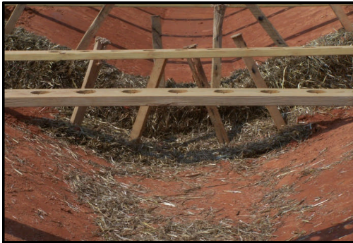
Check Structure Installation over Bare Soil
