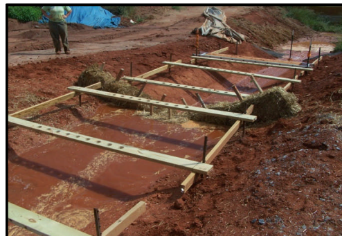
Initial Flow & Upstream Ponding with Some Underflow
