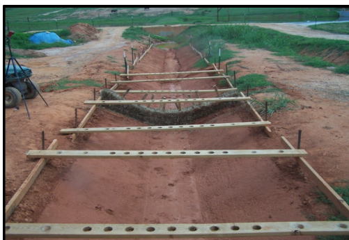
Check Structure Installation over Bare Soil
