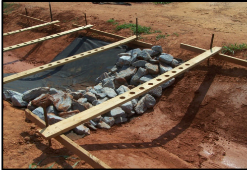
Check Structure Installation over Bare Soil
