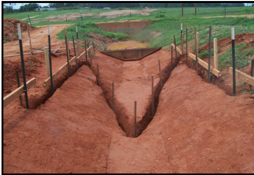
Check Structure Installation over Bare Soil
