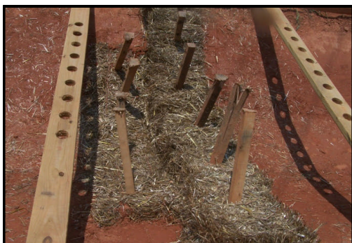
Check Structure Installation over Bare Soil
