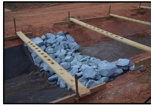
Increased Ponding and Seepage
