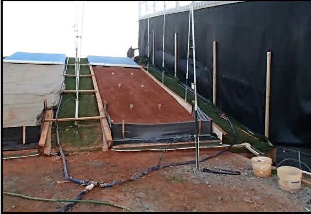
Test Slope Prepared and Fence Installed
