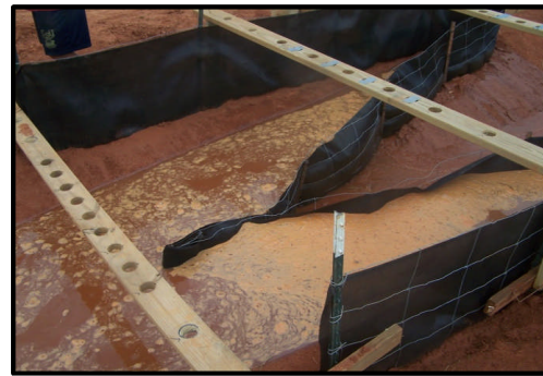
Increased Ponding & Very Near Overtopping
