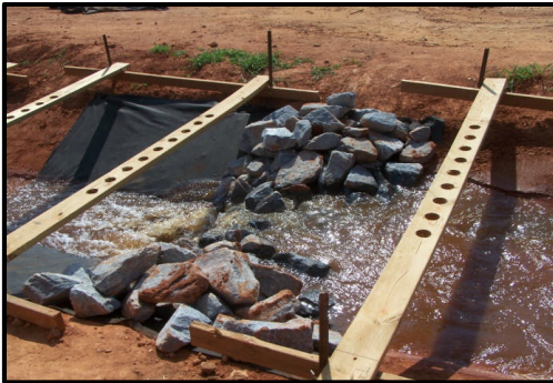
Increased Ponding and Overtopping
