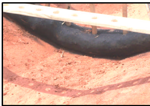
Check Structure Installation over Bare Soil
