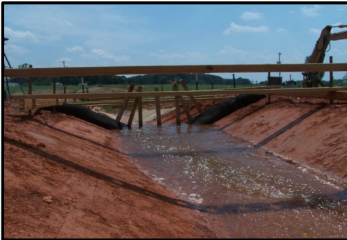
Increased Ponding and Overtopping. No Apparent Underflow
