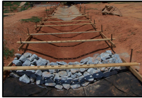
Check Structure Installation over Bare Soil
