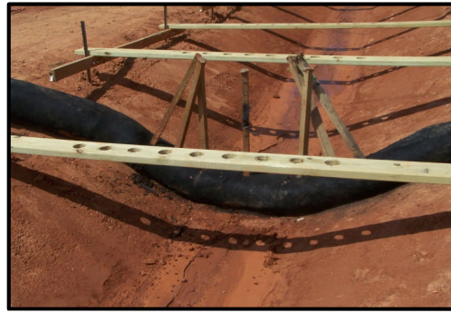
Check Structure Installation over Bare Soil
