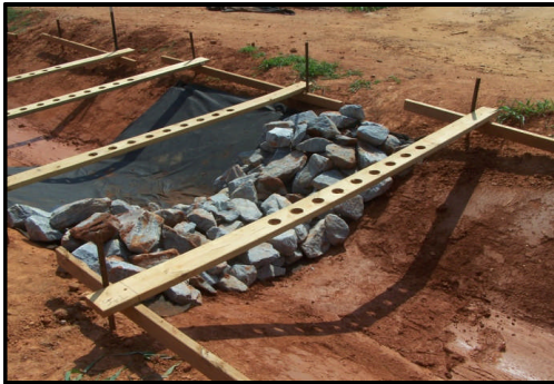
Check Structure Installation over Bare Soil
