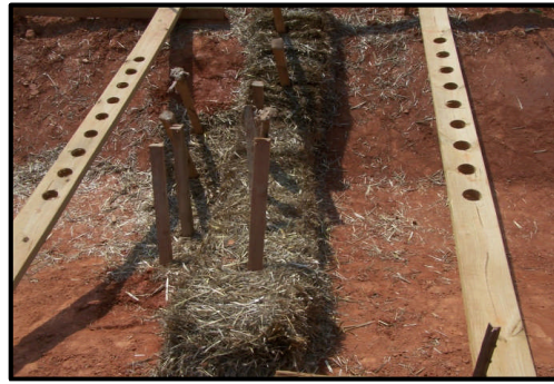
Check Structure Installation over Bare Soil
