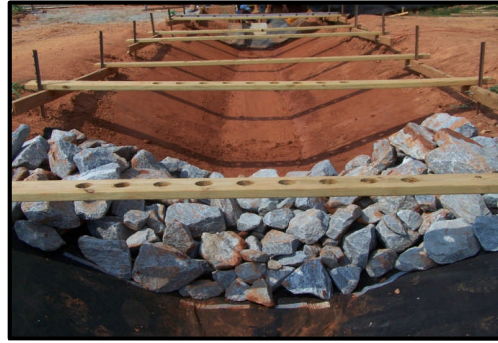
Check Structure Installation over Bare Soil
