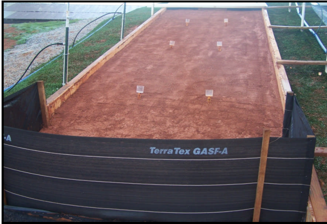
Test Slope Prepared and Fence Installed
