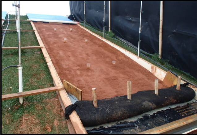
Slope Prepared and Compost Sock Installed
