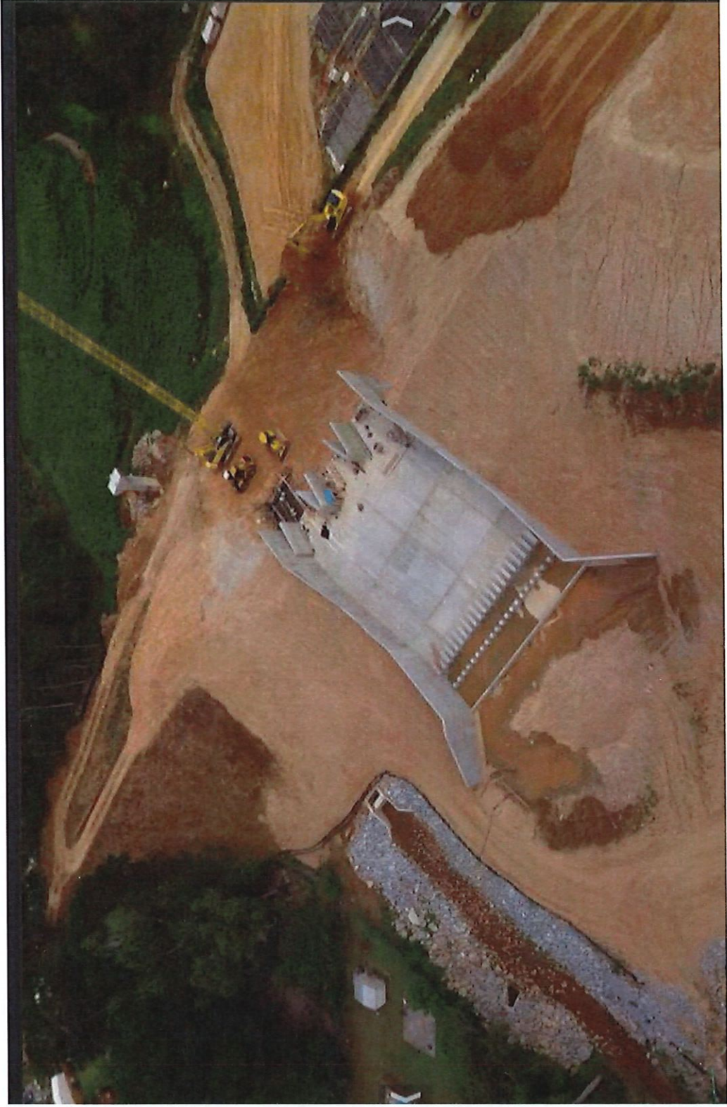
Bull Creek #12 Muscogee County Wing and Labyrinth Wall Progress 6.09.2023
