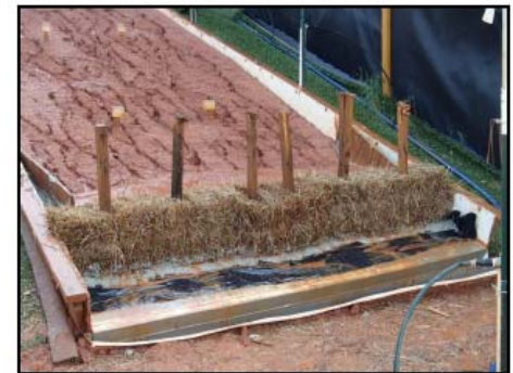
Figure 12. Type B Straw Bales End-of-Test
