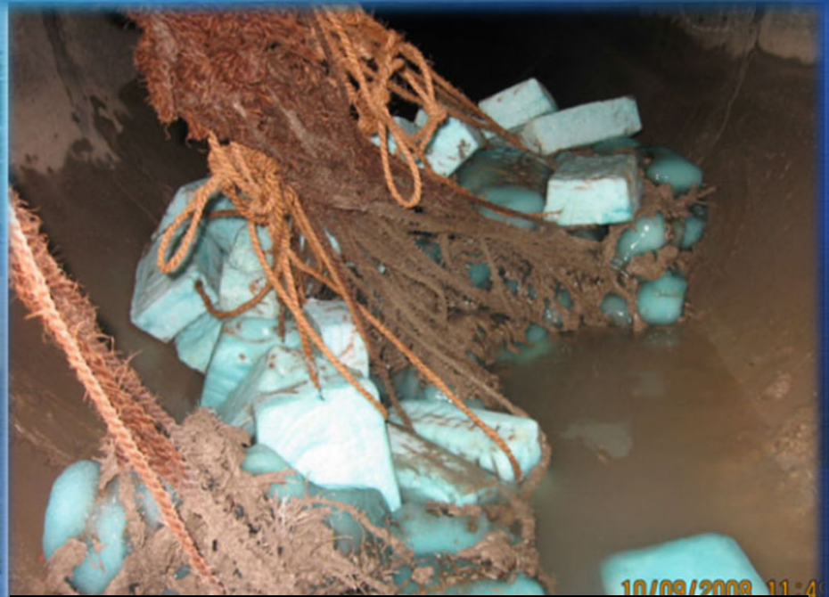
Flocculant Logs Placed In 66" Pipe
