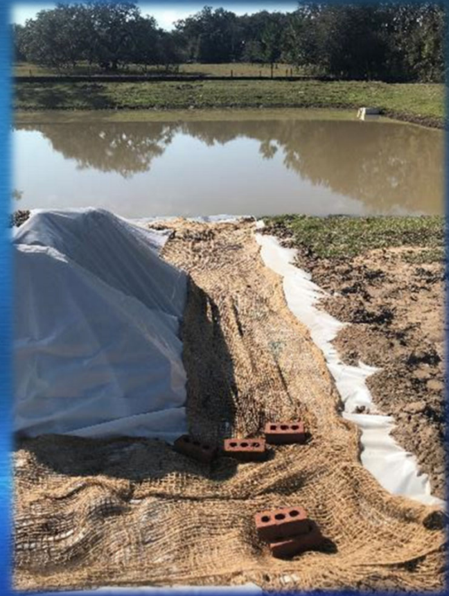
Particle Capture w/Jute
