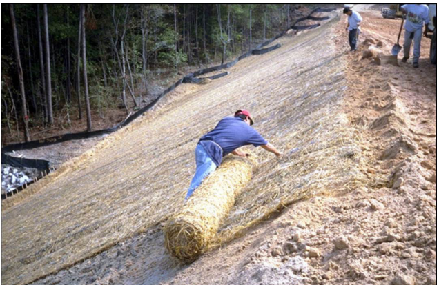
Figure 2. Installation of Jute Matting
