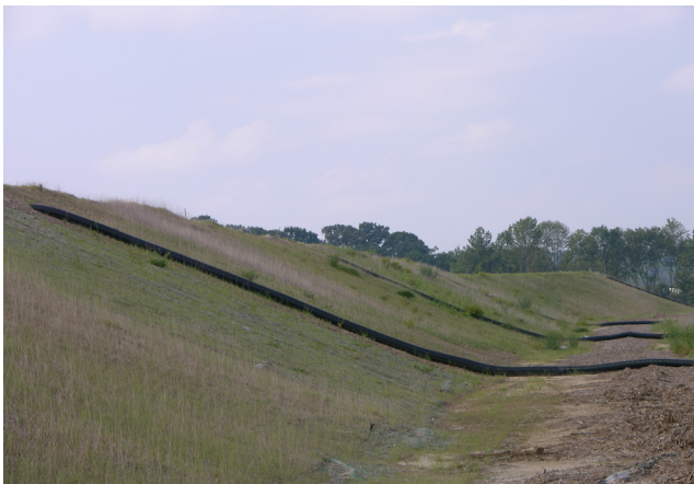
Figure 2. Diagonally Placed Downdrain
