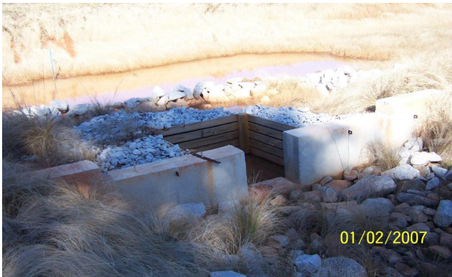
Figure 3. Slotted Board Dam
