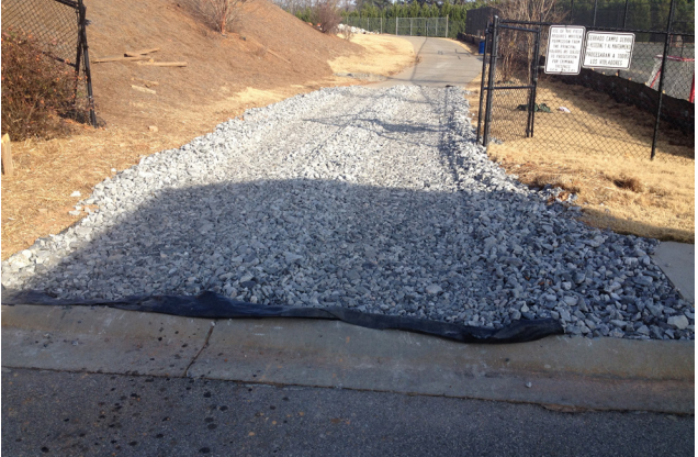
Figure 2. Geotextile Underliner
