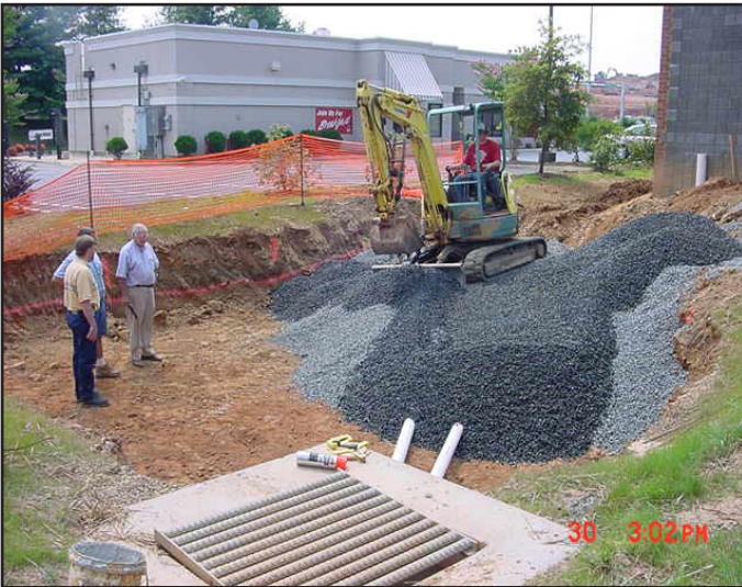
Conversion of a small-scale sediment trap to bioretention. The photos shows adding an under-rain system.
