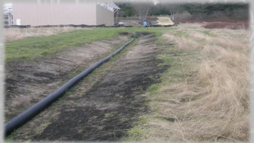
Trenching in wetlands
