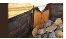
This IECA Design Standard is intended to guide designers on the purpose, design, material selection, installation, and maintenance of a silt fence when used as a temporary sediment control barrier for sheet flow applications to minimize sediment transport from a disturbed area susceptible to erosion.
