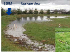
Slow release of water from weep berm outlet to grassed riparian zone.
