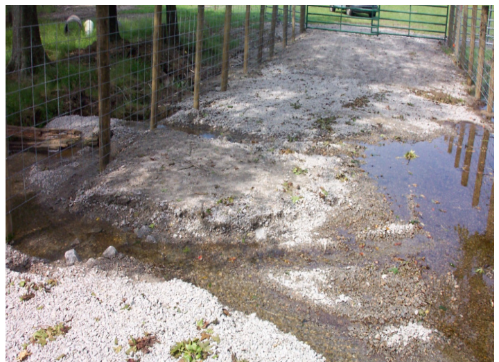
A ford installed as a stream crossing
