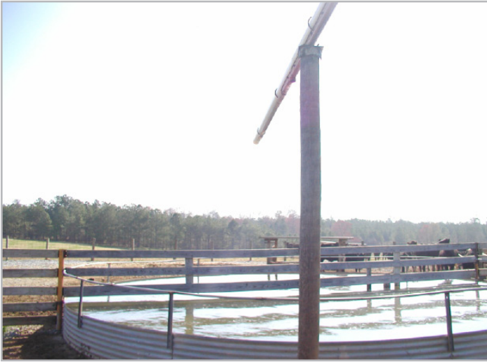
A runoff collection system in Middle Georgia collects rainwater for livestock watering
