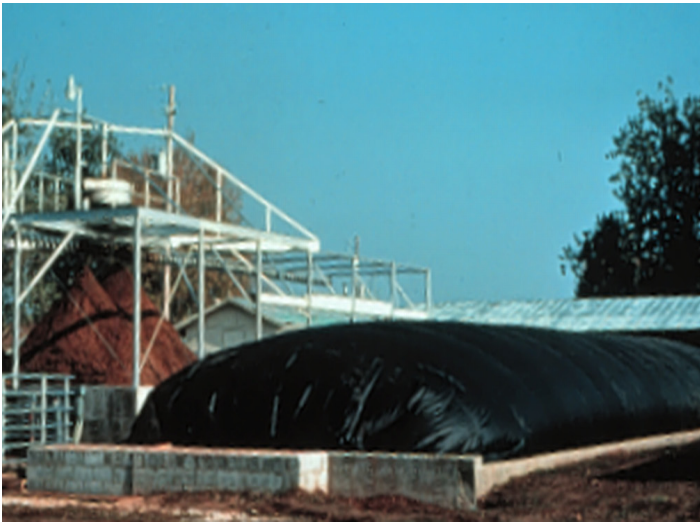
An operational anaerobic digester
