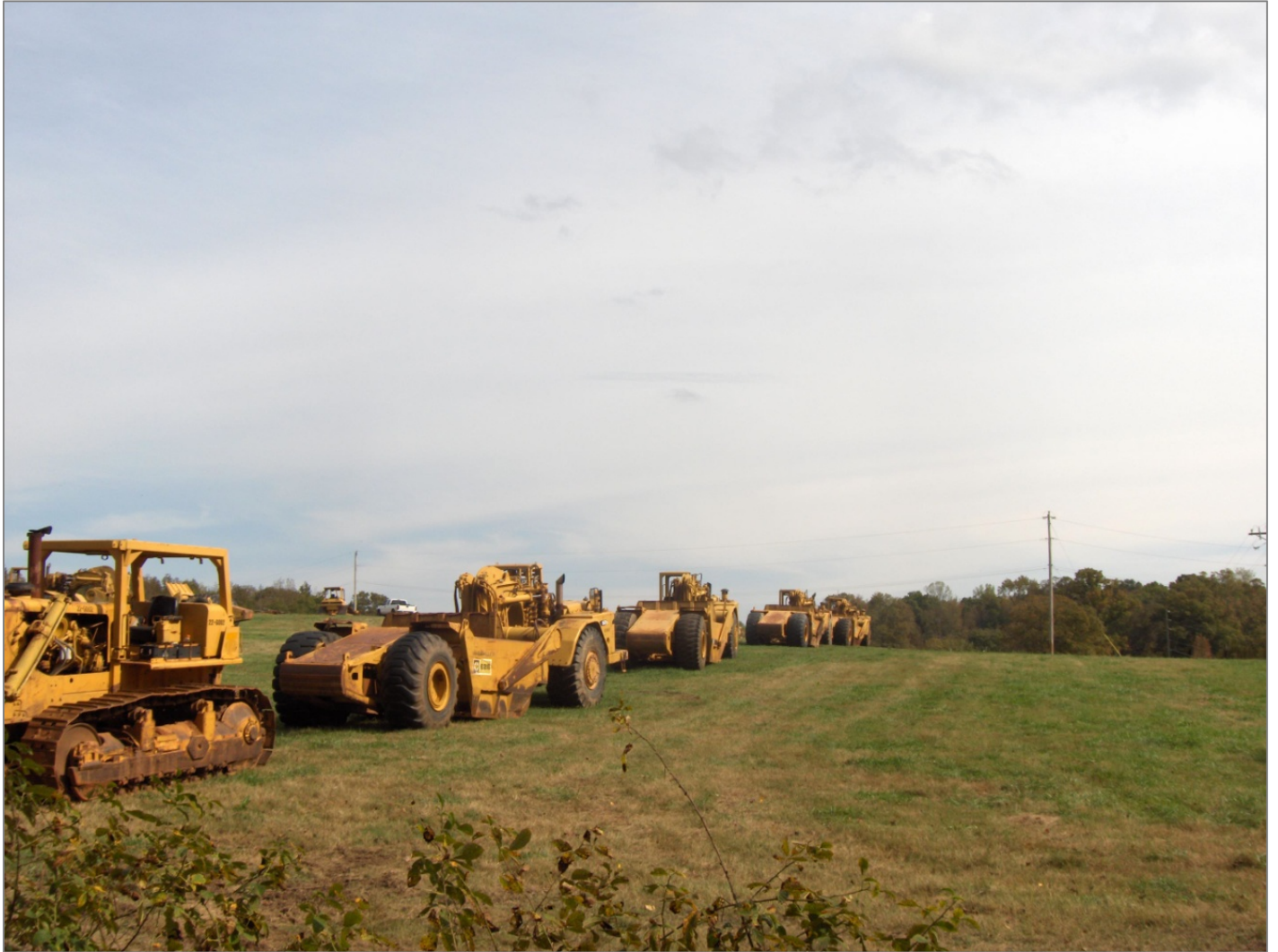
Equipment lined up waiting to begin land grading.
