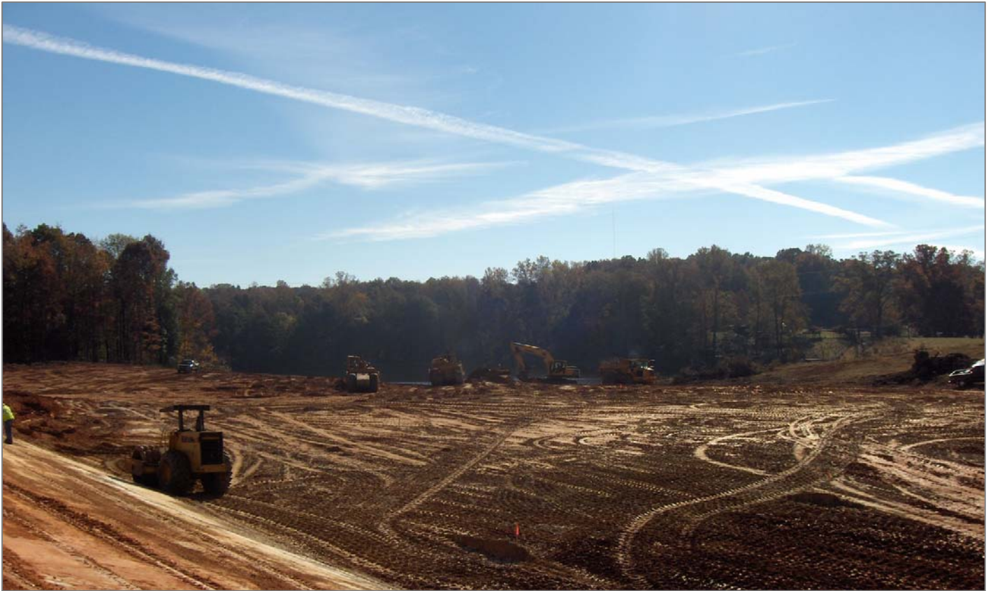
Widening the Spillway
