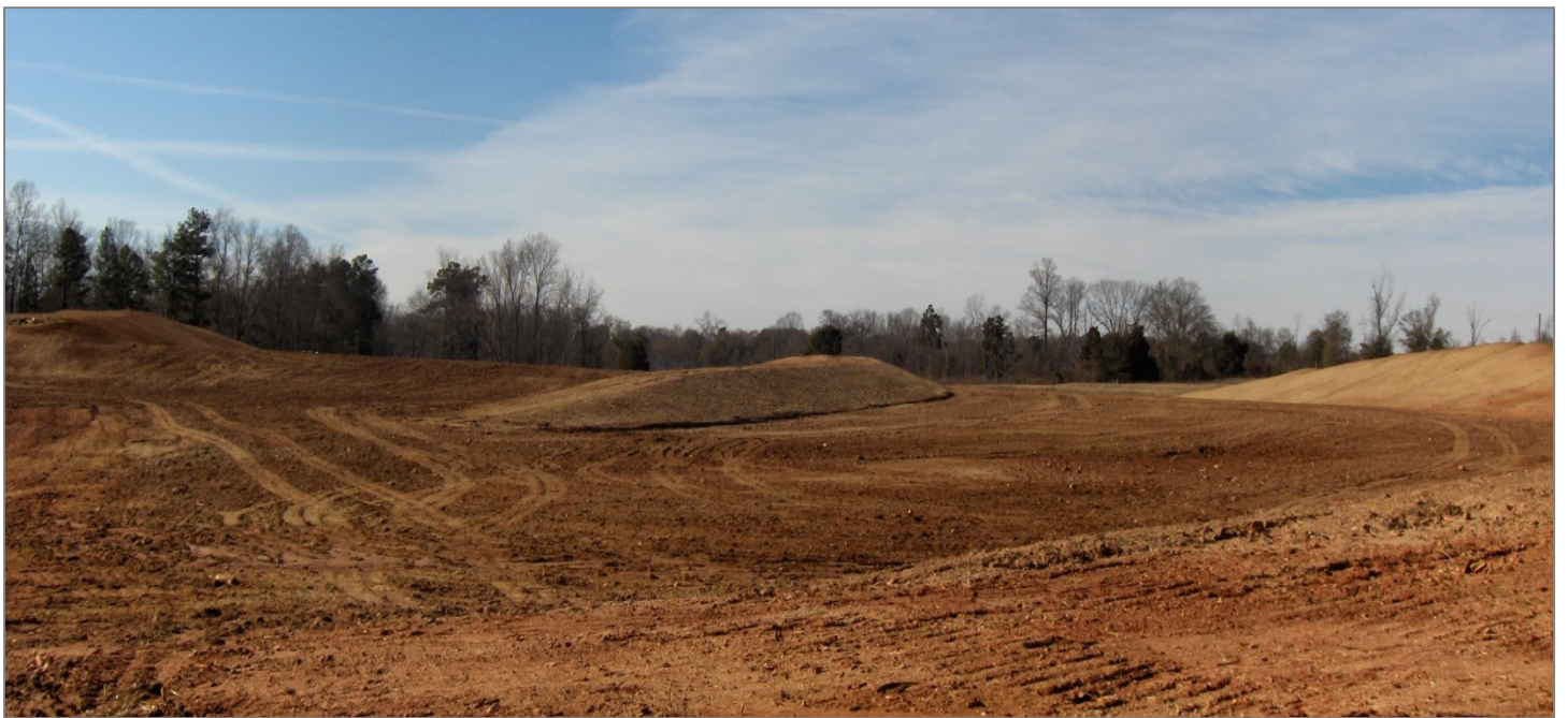
Widening auxiliary spillway with splitter dike.
