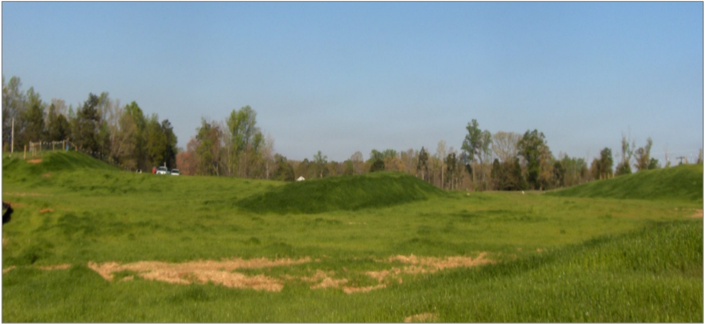
The newly vegetated 300 ft. wide auxiliary spillway with 40 ft. splitter dike.
