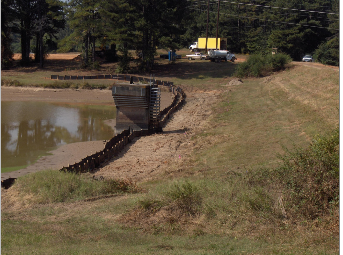
Preconstruction on Marbury Creek #22
