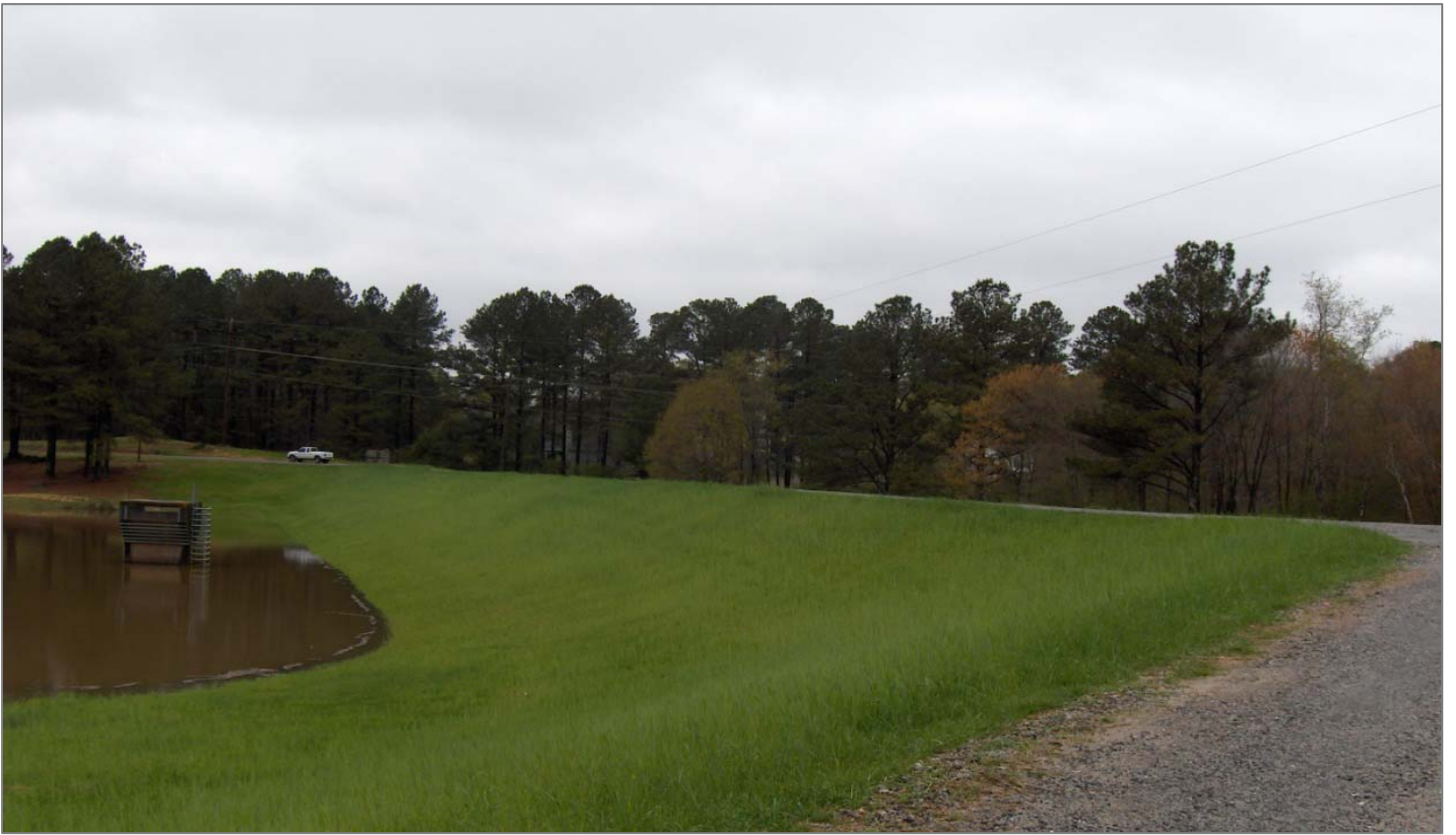
The newly vegetated front slope and spillway.
