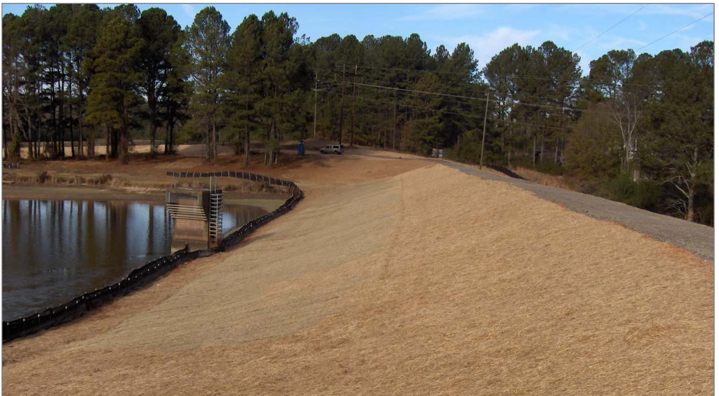
The slope is seeded and mulched.
