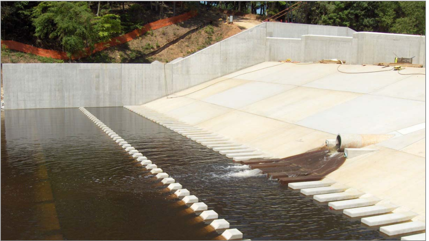
June 2011 - The completed working end of the new auxiliary spillway
