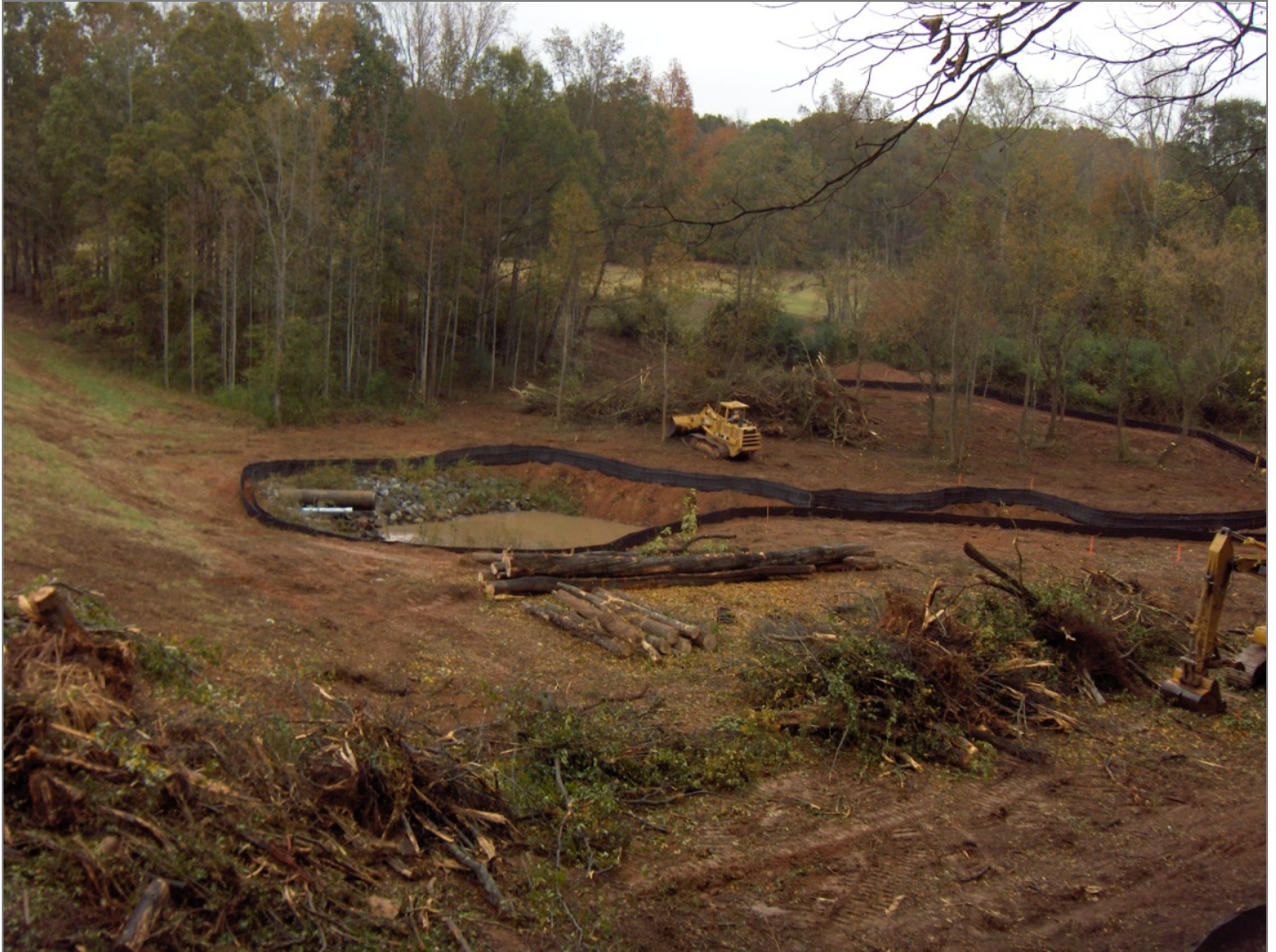
November 2010 - Vegetation is cleared around the plunge pool
