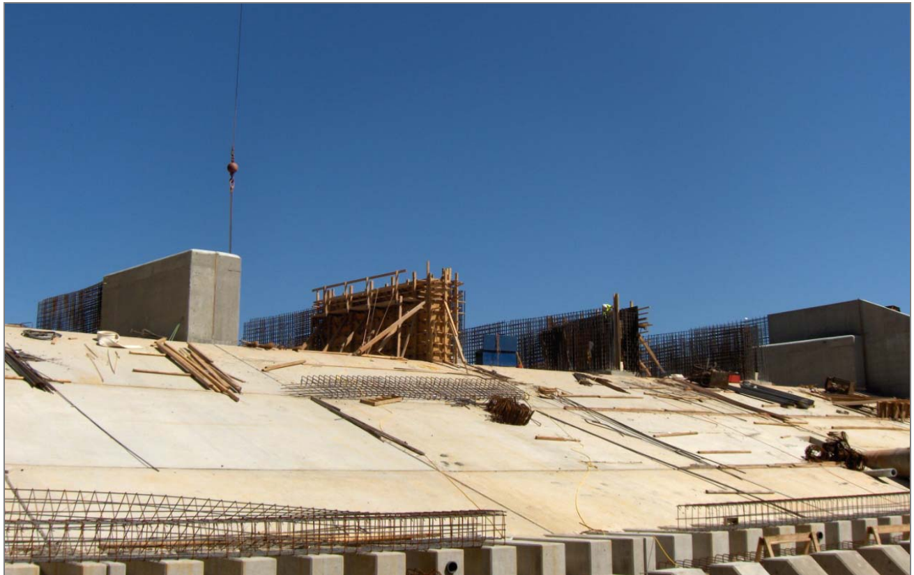
April 2011 - Forming the weir walls
