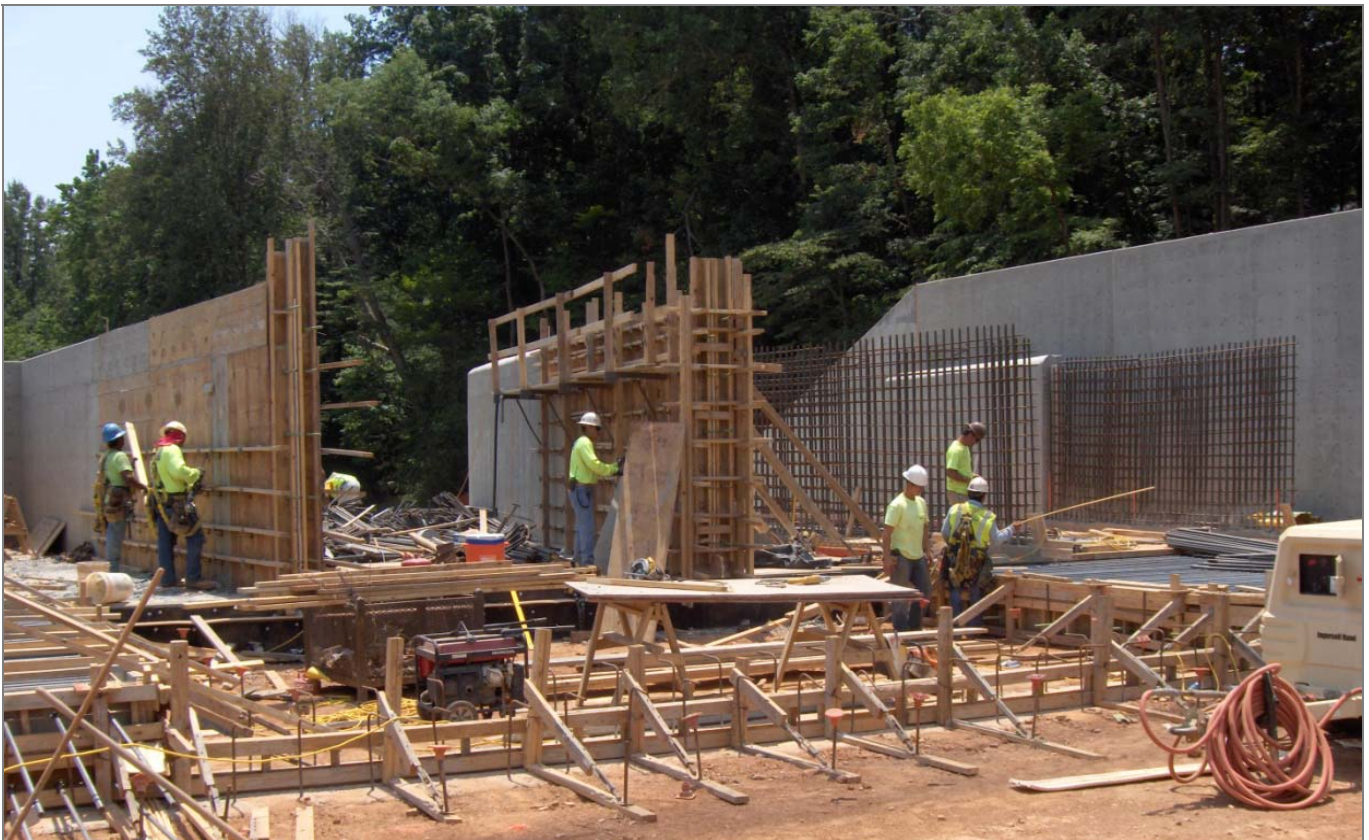
Weir wall construction seen from the front side of the dam.
