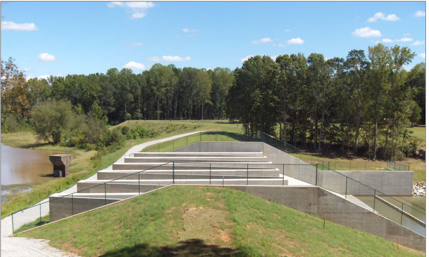
September 2011 – View overlooking the completed dam from the side
