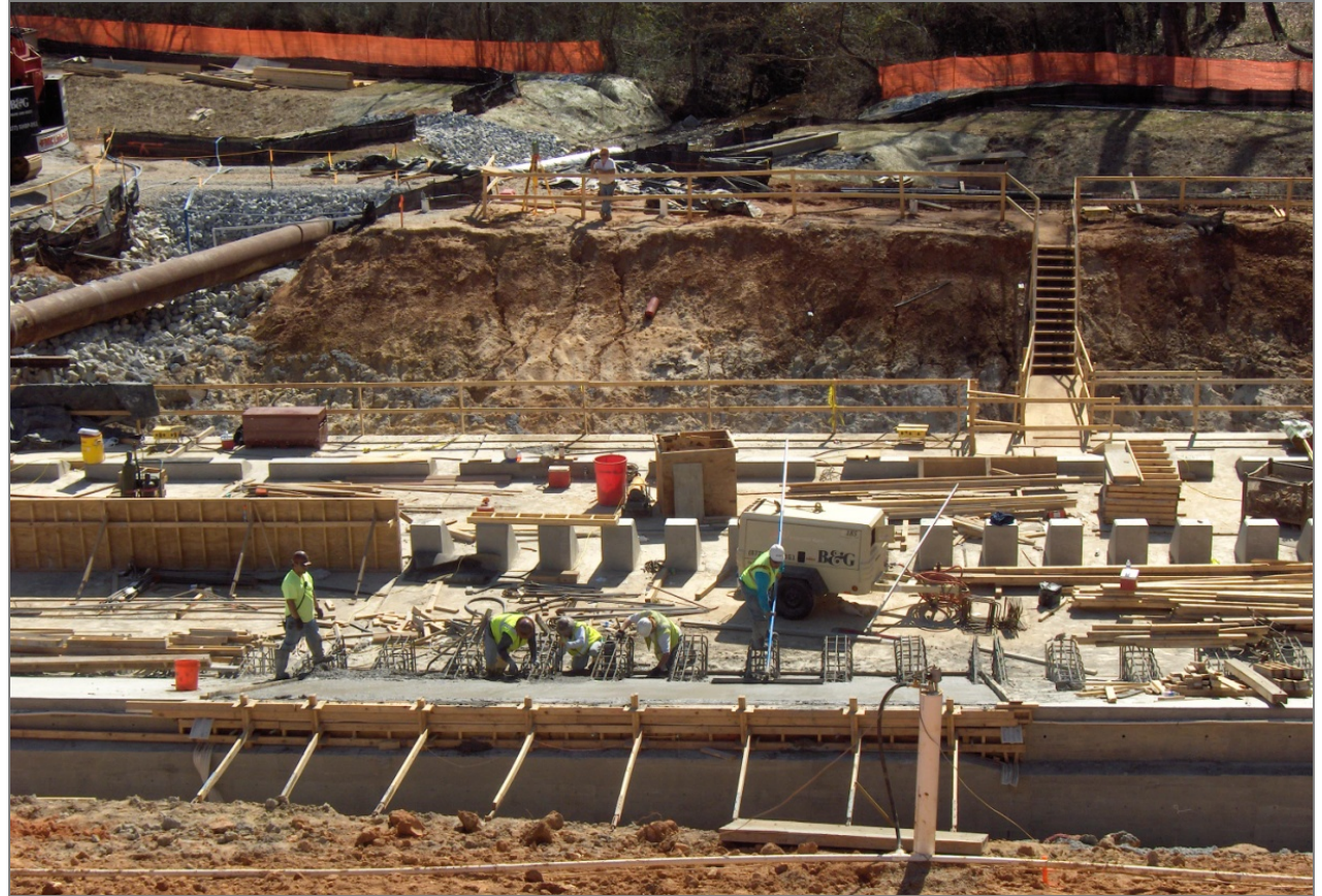
February 2011 - Spillway construction is ongoing
