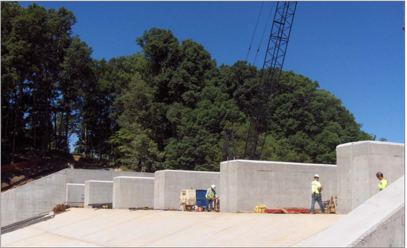
May 2011 - A view of the weir walls from the backside of the dam.
