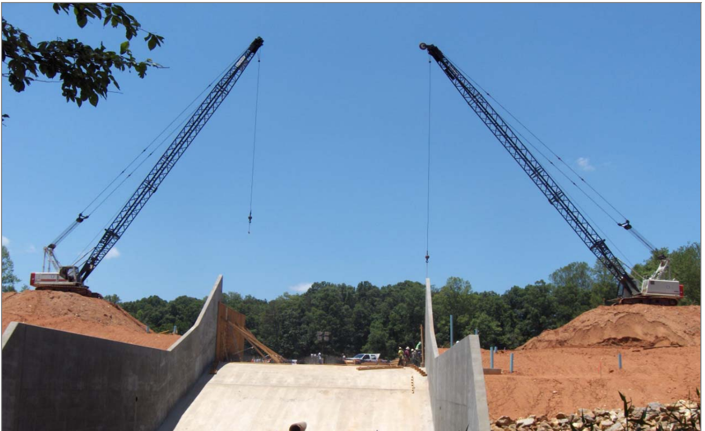
View of the new chute spillway
