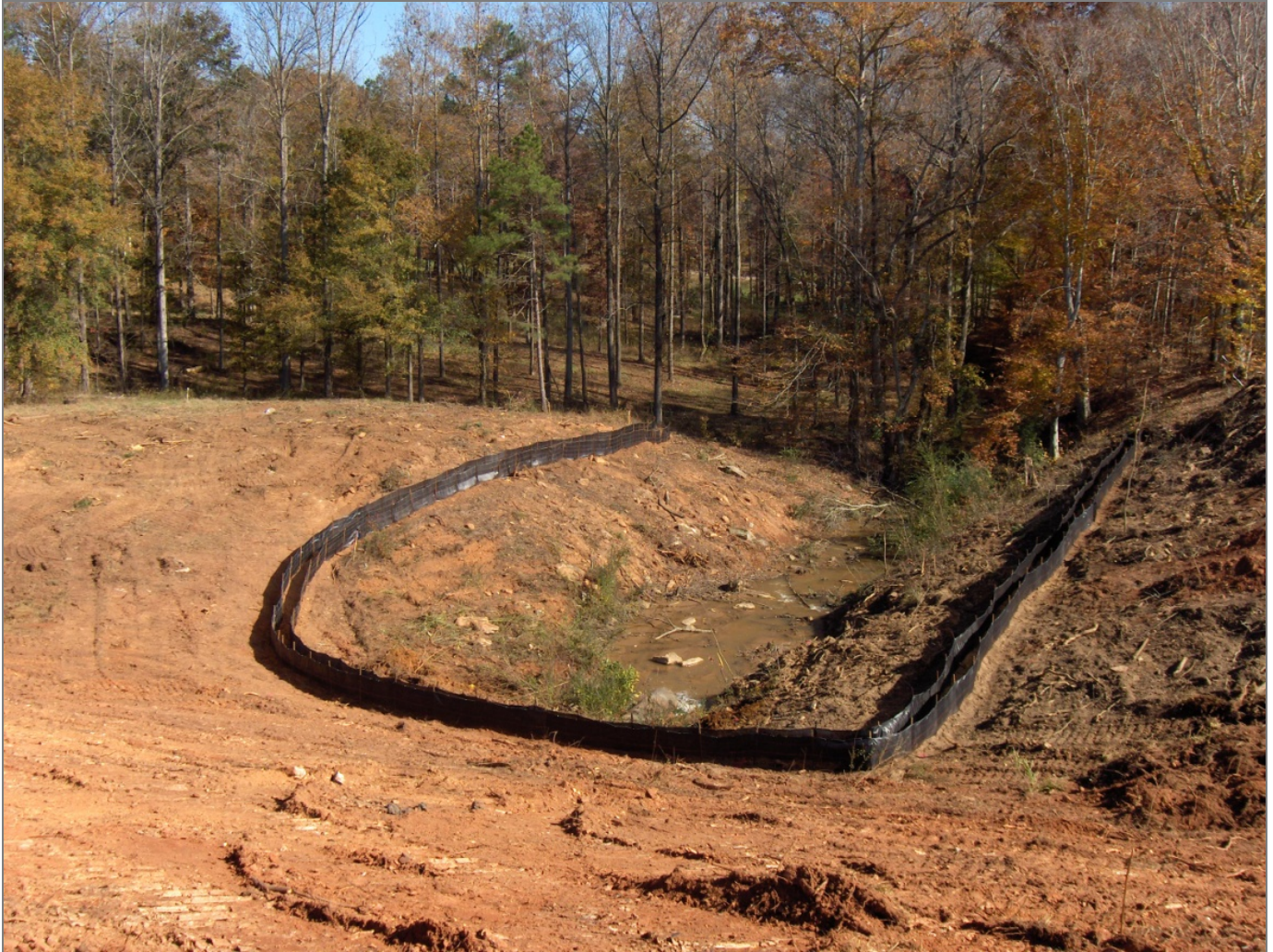
December 2010 - Clearing and regrading of back slope & spillway
