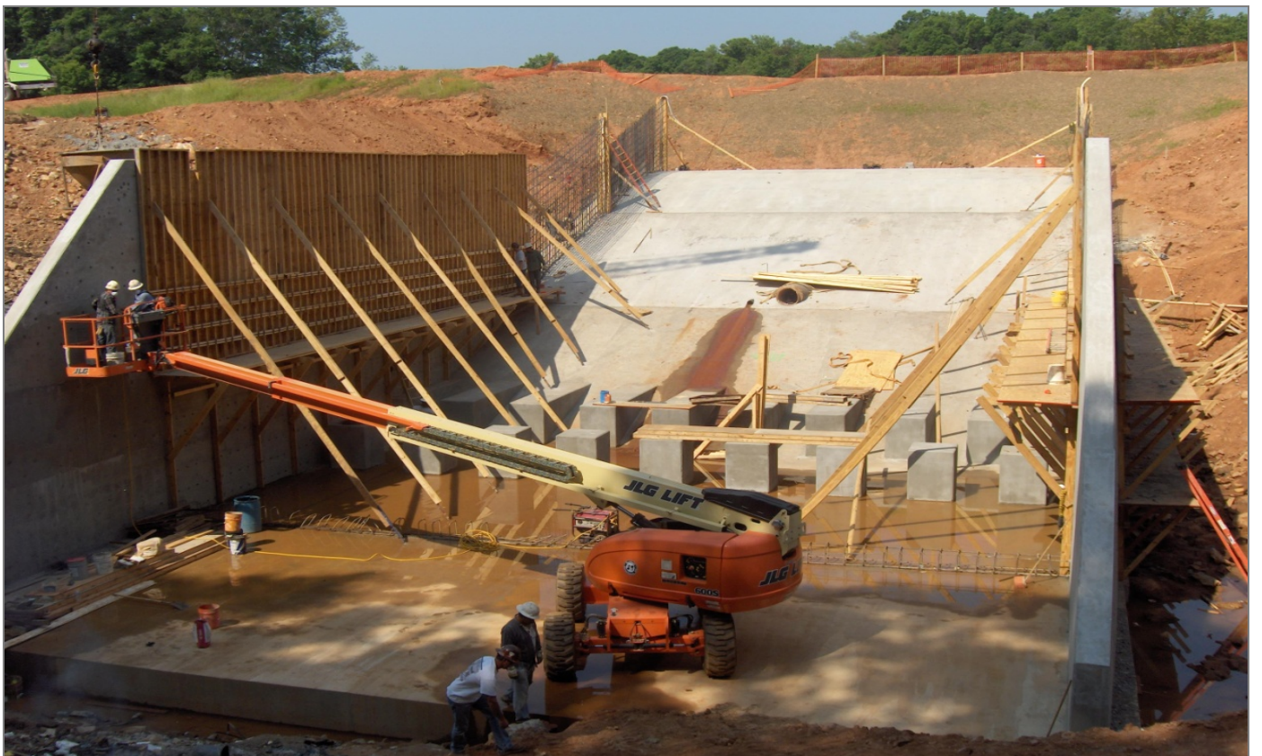
May 2011 - Forming the spillway walls
