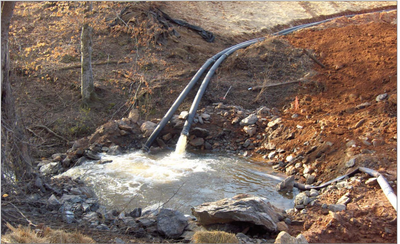
February 2011 - Water is rerouted during spillway construction
