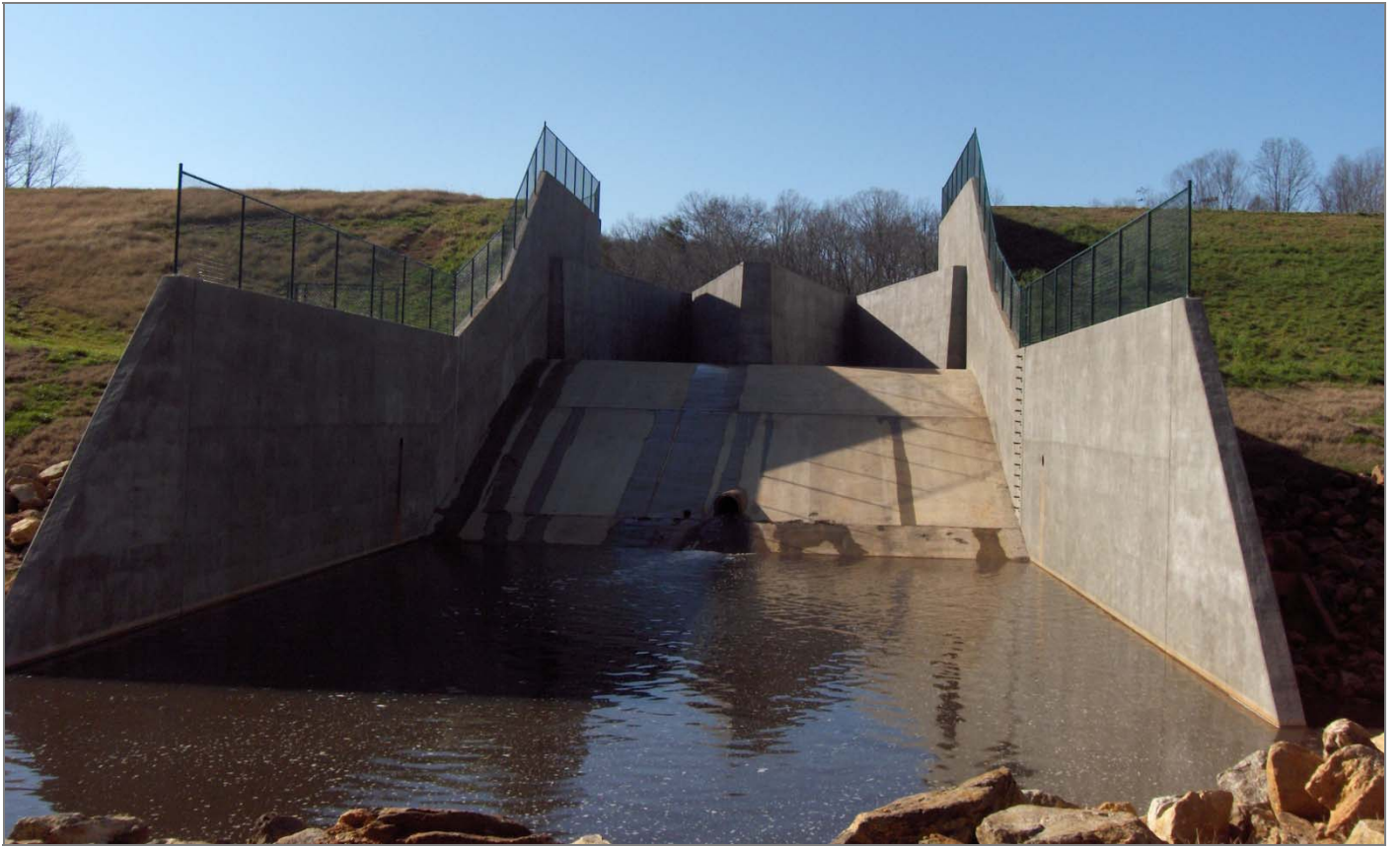
The completed spillway
