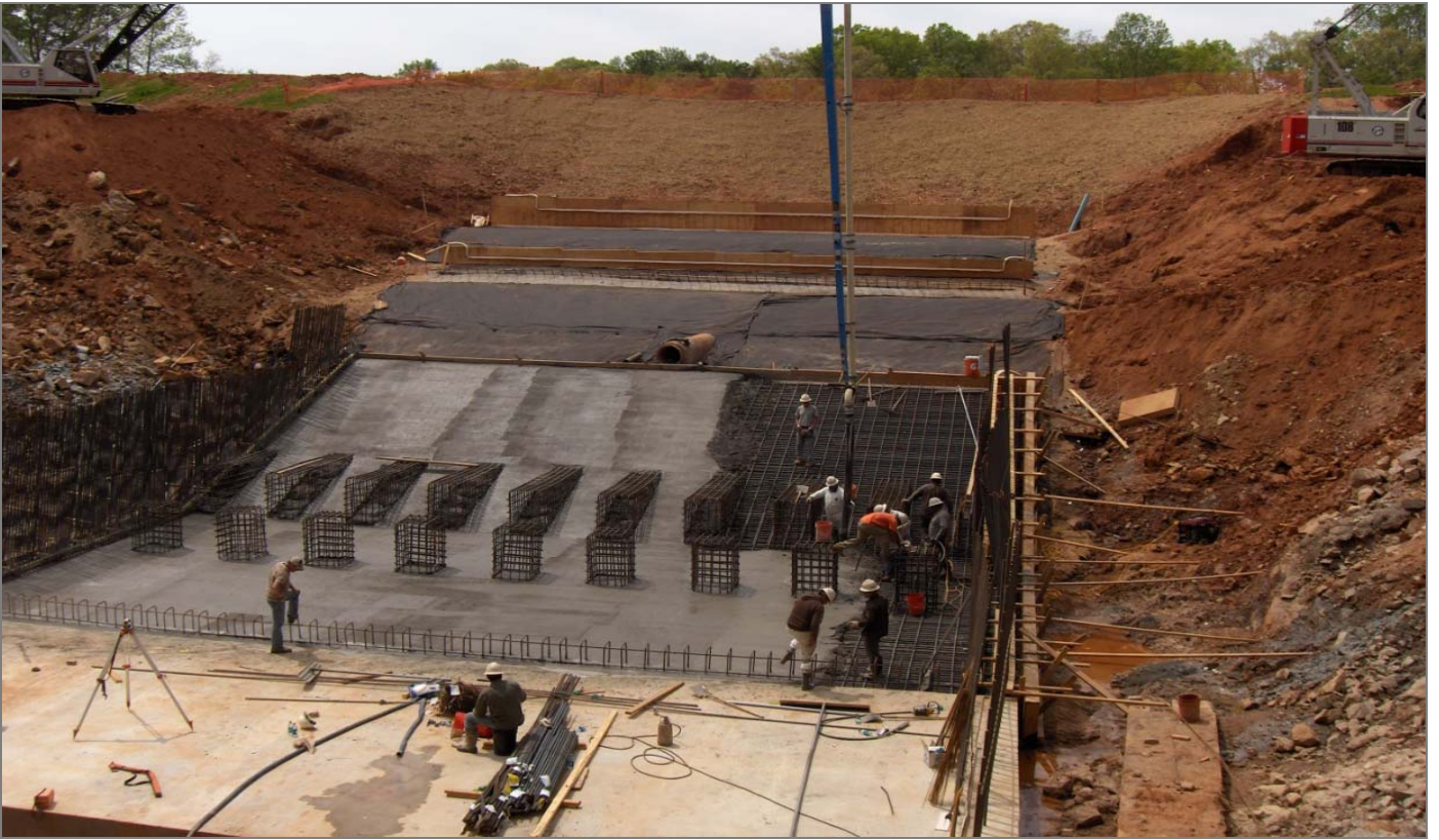
April 2011 - Pouring a section of the chute spillway
