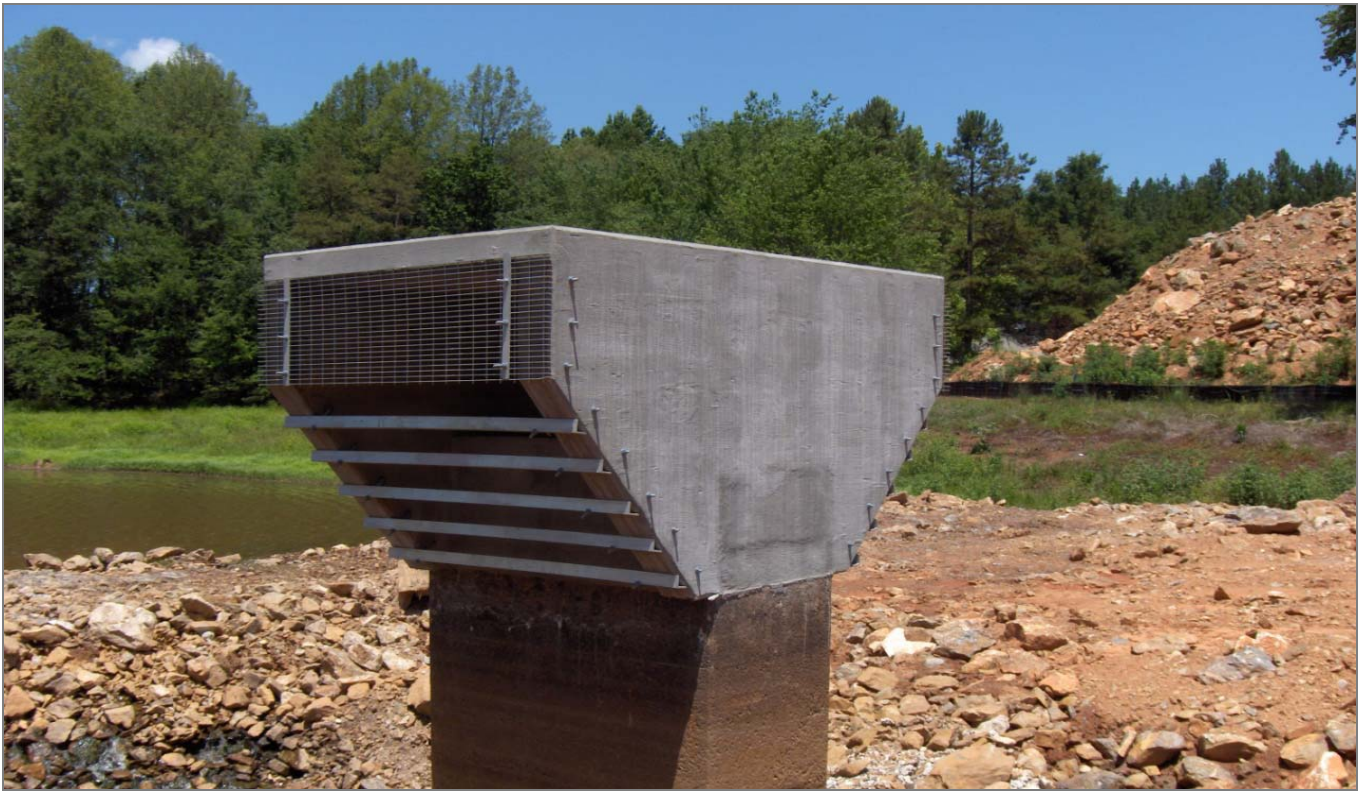
June 2011- The new principle spillway riser
