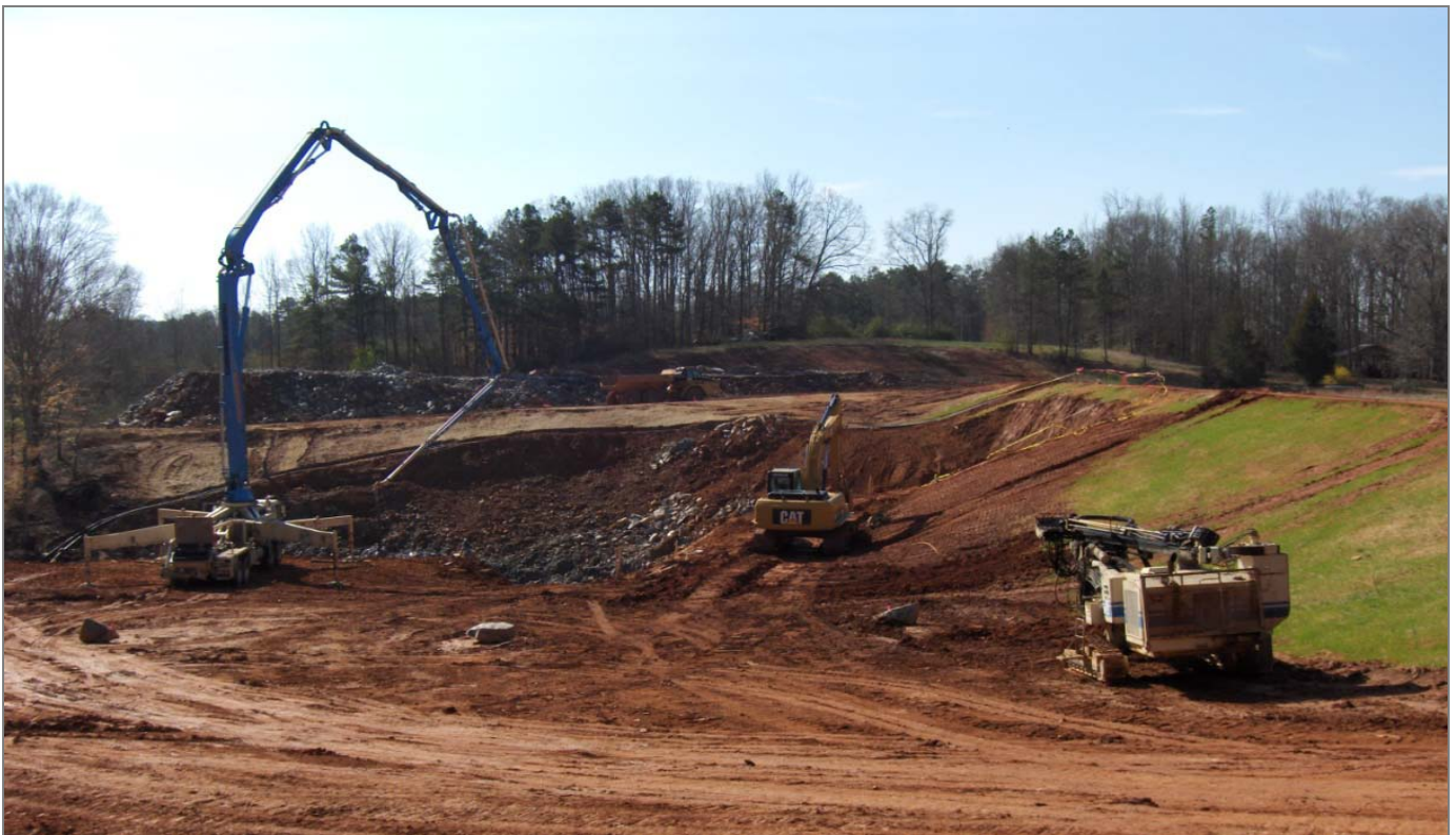
March 2011 - Excavation of chute area behind South Fork Dam #4
