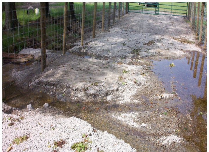
A ford installed as a stream crossing
