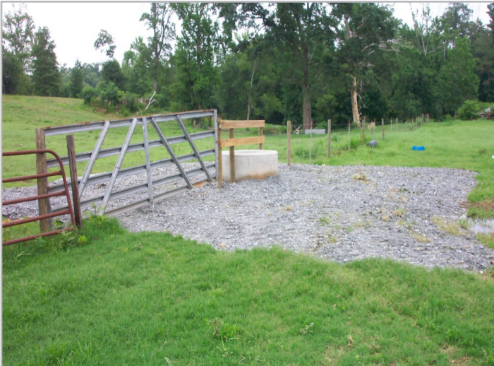
Heavy Use Area Protection around a watering trough
