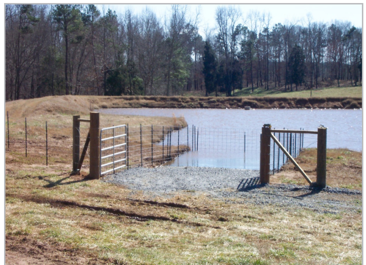
A watering ramp with fencing to limit access
