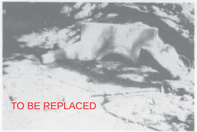
Figure 1-3. - Sediment from upstream erosion has severely reduced the capacity of this culvert.
