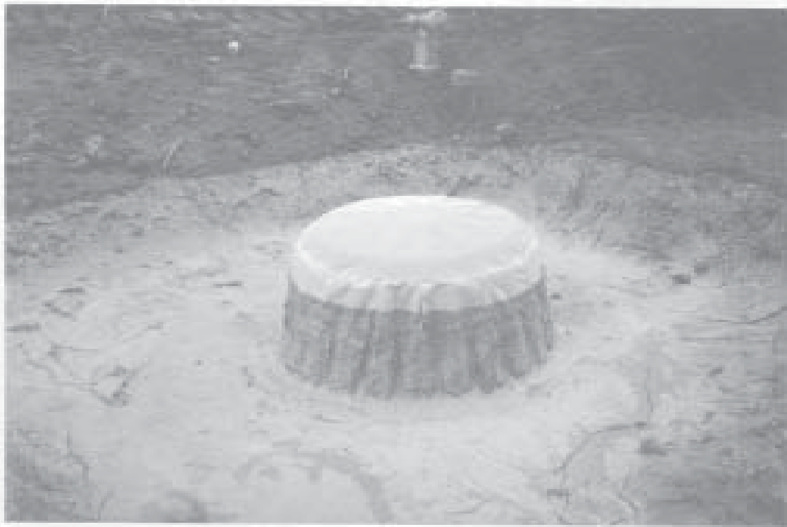
Figure 6-21.7 - Alternative Inlet Sediment Trap
