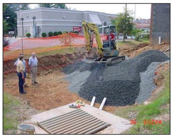
Conversion of a small-scale sediment trap to bioretention. The photos shows adding an underd-rain system.
