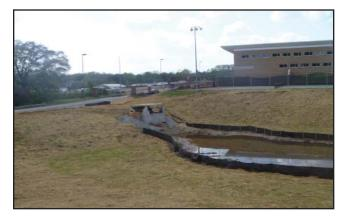
Figure 2.11 - This temporary sediment basin effectively trapped sediment from upstream erosion.
