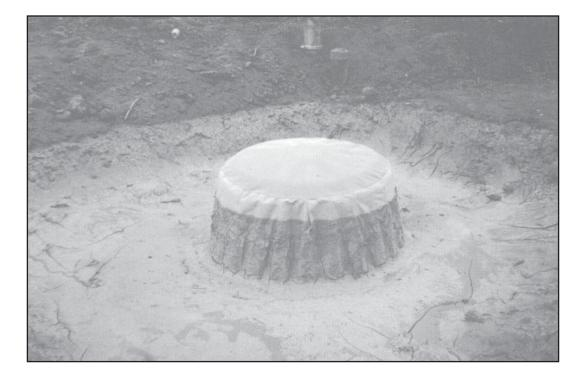
Figure 6-28.7 Alternative Inlet Sediment Trap
