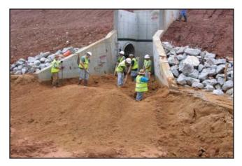
Figure 1.2 - Maintaining outlet protection due to BMP failures higher in the drainage basin.
