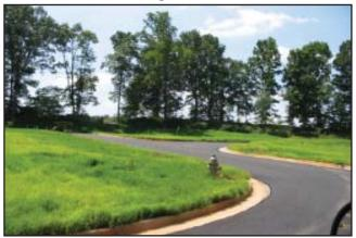
Figure 2.6 - Vegetation on this road bank will reduce erosion to a minimum.
