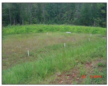
Conversion of a sediment basin to a bioretention area. The original riser acts as the overflow structure for the bioretention practice.
