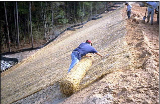
Figure 2. Installation of Jute Matting
