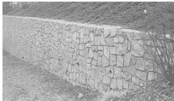
Figure 1. Typical Stone Retaining Wall
