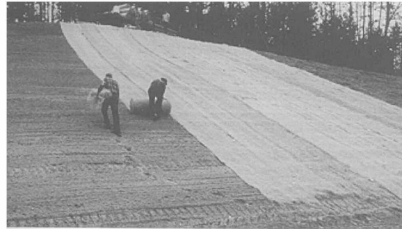
Figure 1. Installation of Jute Matting
