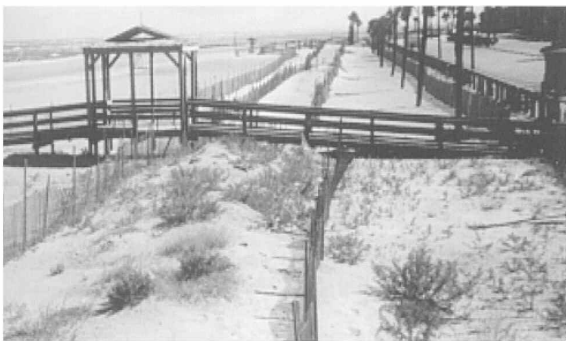
Figure 1. Sand Fence and Native Plants
