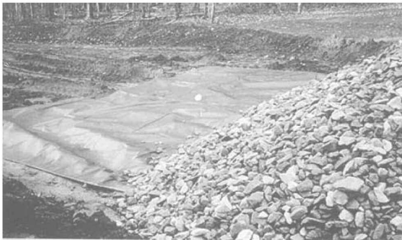
Figure 2. Geotextile Underliner Under Gravel Pad
