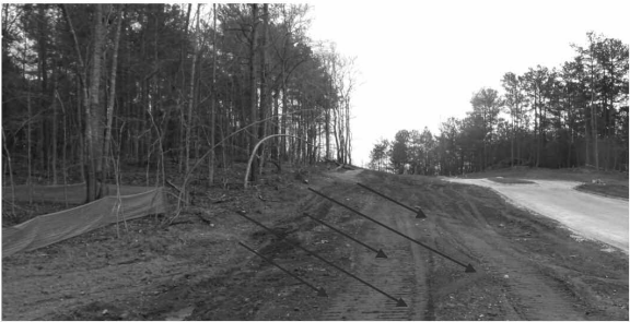
Sheet Erosion: Erosion caused by water flowing in a thin layer over the ground surface
