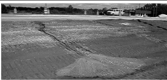
Rill Erosion: An erosion process in which numerous small channels only several inches deep are formed
