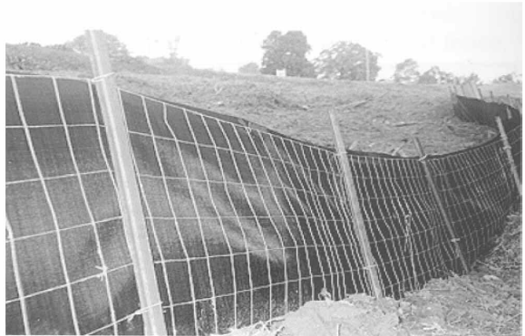
Figure 5. Typical Type "C" Silt Fence
