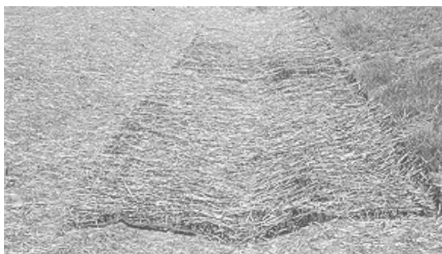
Figure 2. Geotextile Installed to Control Erosion in a Concentrated Flow Area
