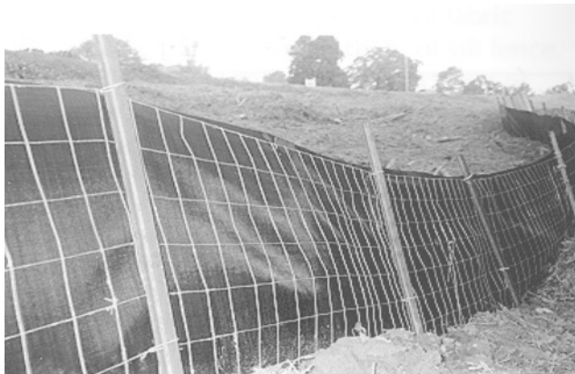
Figure 5. Typical Type “C” Silt Fence
