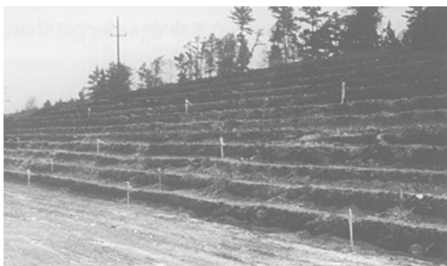
Figure 2. Typical Stair-Step Grading
