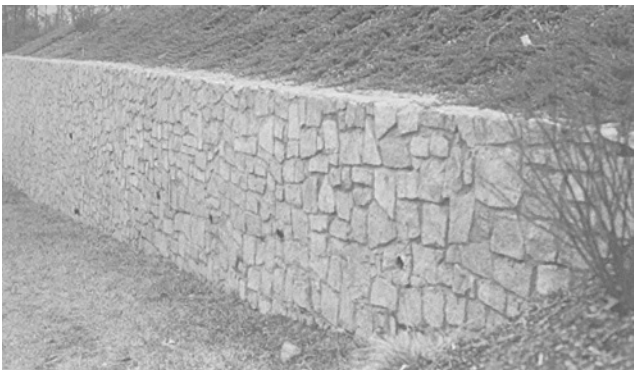
Figure 1. Typical Stone Retaining Wall
