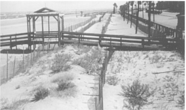
Figure 1. Sand Fence and Native Plants
