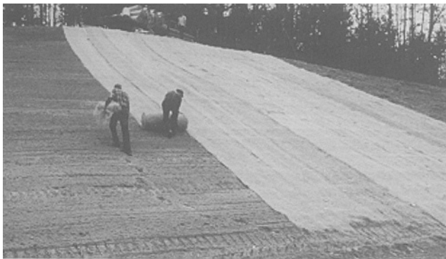
Figure 1. Installation of Jute Matting
