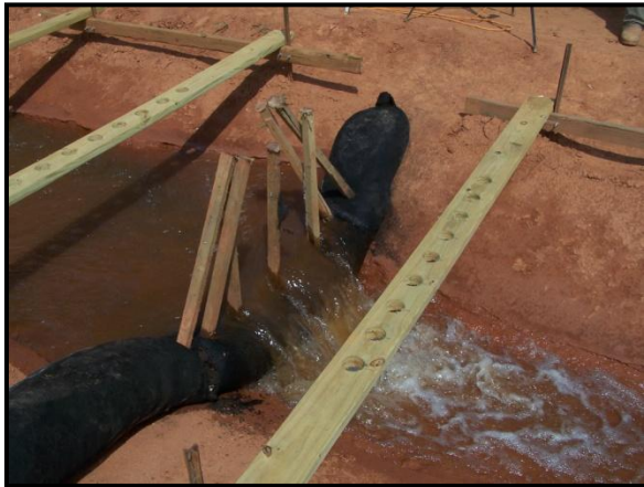
Figure 21. Compost Sock Check Structure
