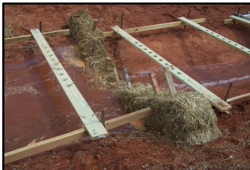
Increased Ponding, Start Overtopping, Increased Underflow
