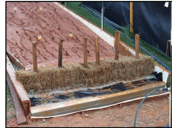
Figure 12. Type B Straw Bales End-of-Test
