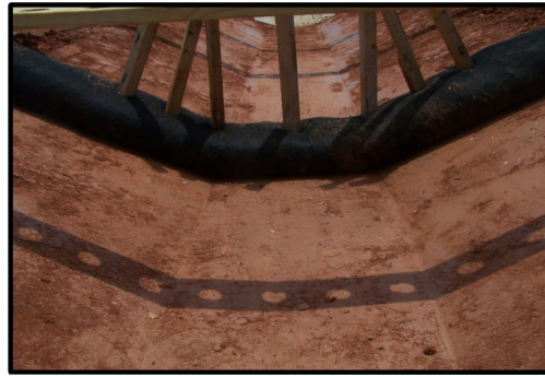
Check Structure Installation over Bare Soil
