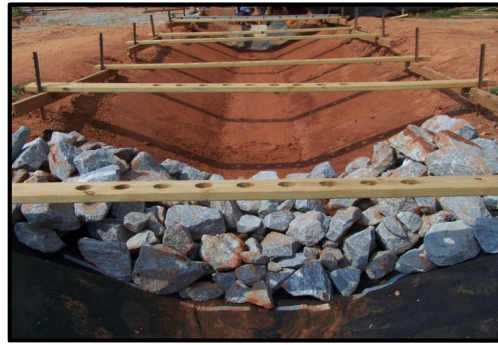
Check Structure Installation over Bare Soil
