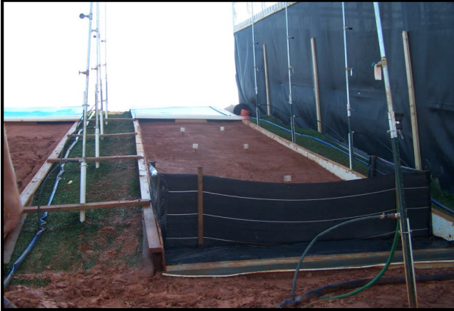
Test Slope Prepared and Fence Installed
