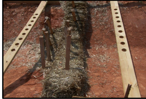
Check Structure Installation over Bare Soil
