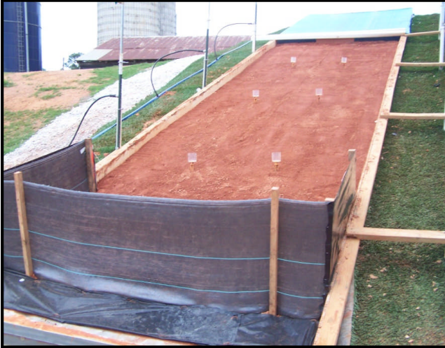
Test Slope Prepared and Fence Installed
