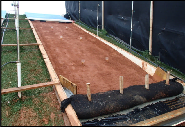
Slope Prepared and Compost Sock Installed
