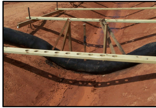
Check Structure Installation over Bare Soil
