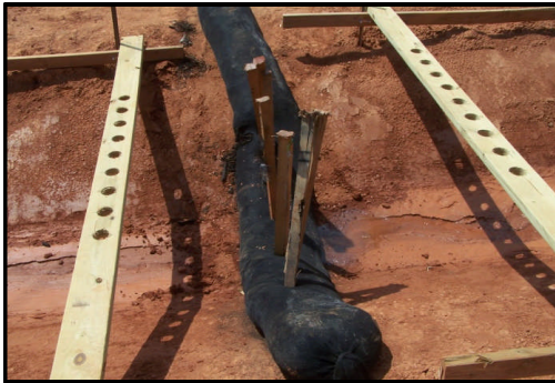
Check Structure Installation over Bare Soil
