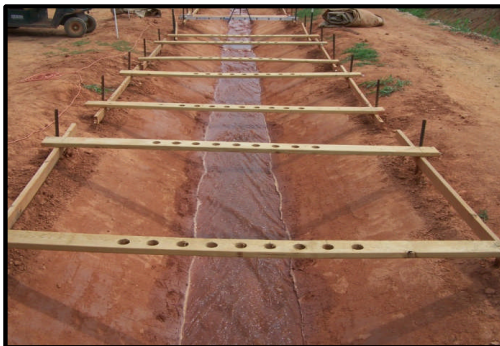
Initial Flow & Inlet Weir
