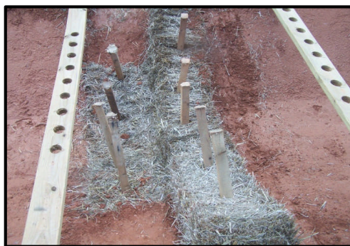
Check Structure Installation over Bare Soil
