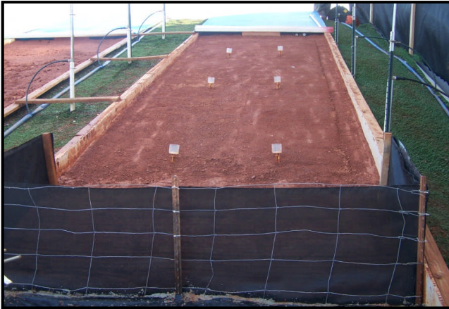
Test Slope Prepared and Fence Installed
