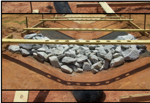
Check Structure Installation over Bare Soil
