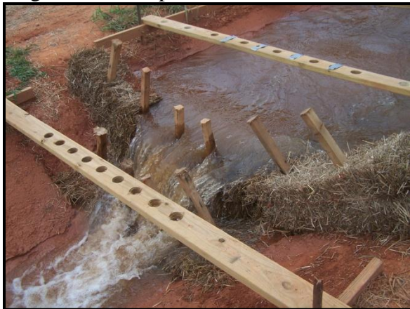
Figure 23. Straw Bale (NRCS) Check Structure
