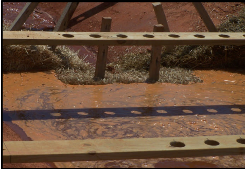
Increased Ponding and Undermining
