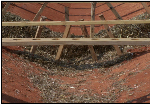
Check Structure Installation over Bare Soil
