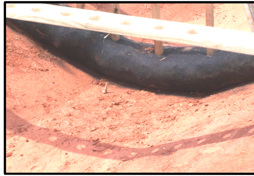
Check Structure Installation over Bare Soil
