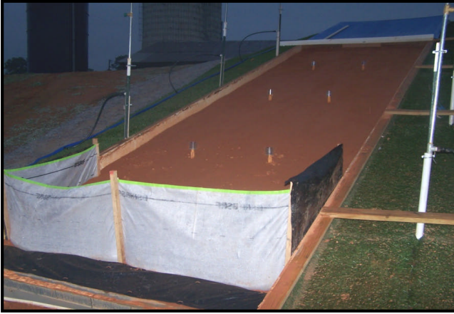
Test Slope Prepared and Fence Installed
