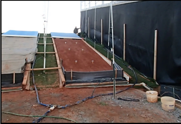
Test Slope Prepared and Fence Installed
