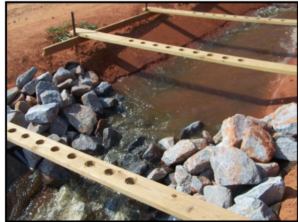
Figure 22. Rock Check Structure
