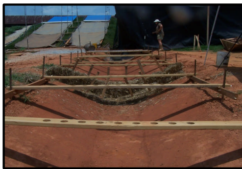
Check Structure Installation over Bare Soil
