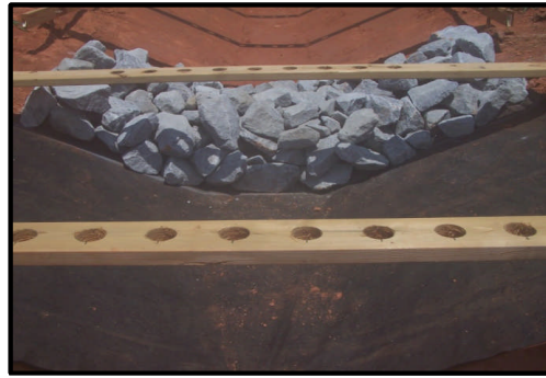
Check Structure Installation over Bare Soil
