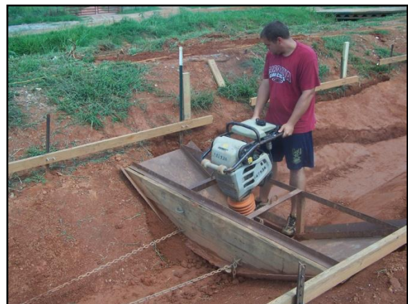
Figure 20. Channel Forming (typical)
