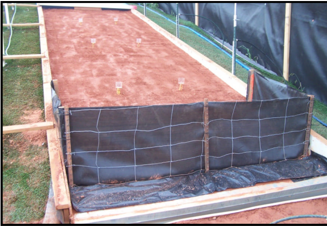
Test Slope Prepared and Fence Installed
