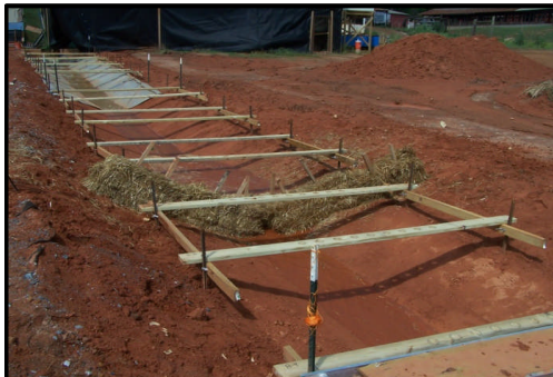
Check Structure Installation over Bare Soil
