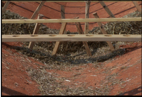
Check Structure Installation over Bare Soil
