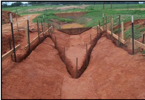
Check Structure Installation over Bare Soil
