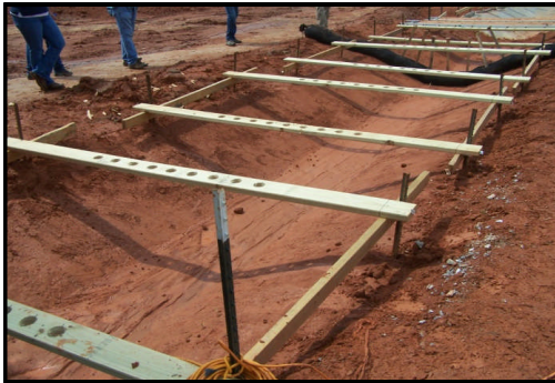
Check Structure Installation over Bare Soil
