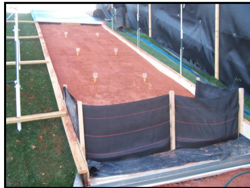
Figure 4 Typical Prepared Slope & Sediment Barrier Installation
