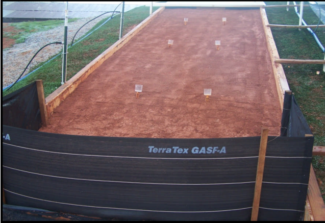
Test Slope Prepared and Fence Installed
