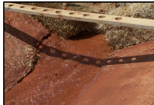
Increased Ponding and Undermining
