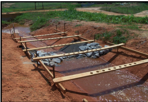
Increased Ponding & Overtopping
