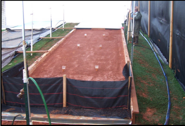
Test Slope Prepared and Fence Installed
