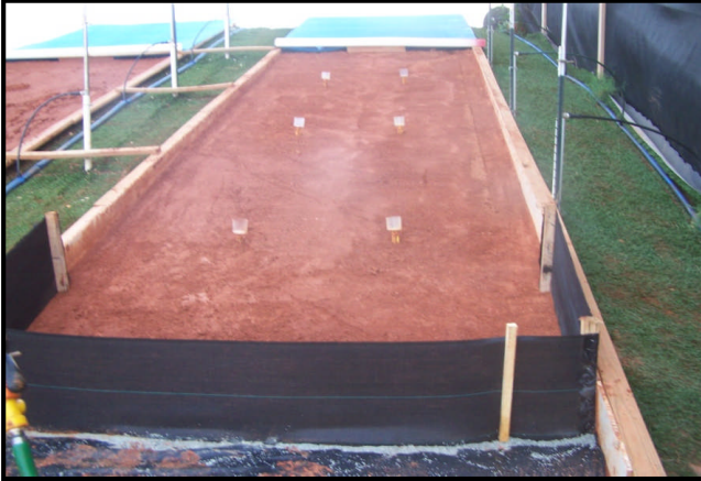
Test Slope Prepared and Fence Installed
