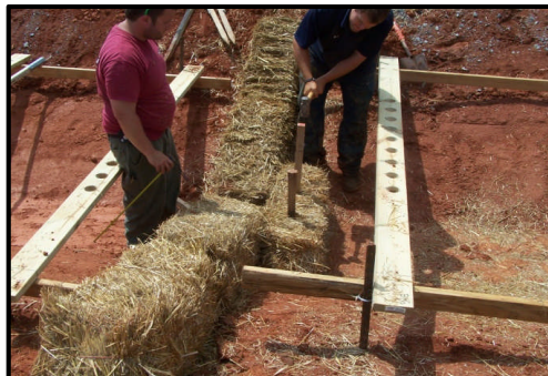
Check Structure Installation over Bare Soil
