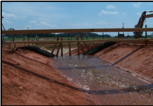
Increased Ponding and Overtopping. No Apparent Underflow
