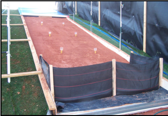
Test Slope Prepared and Fence Installed
