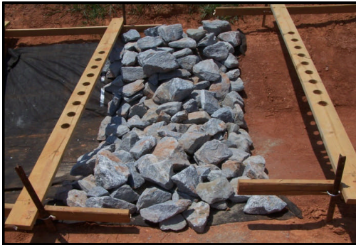
Check Structure Installation over Bare Soil
