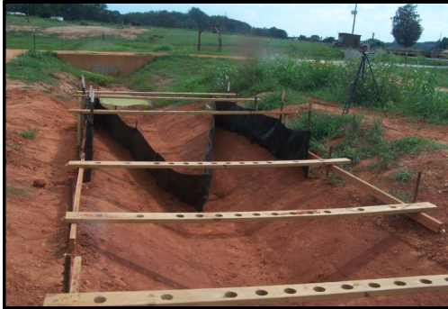
Check Structure Installation over Bare Soil
