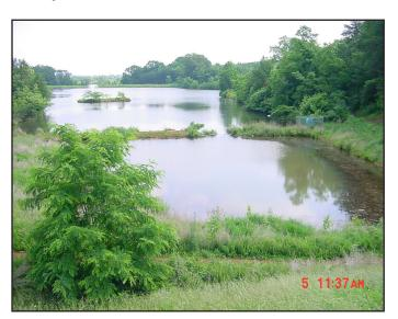
Post-construction conversion called for the creation of sediment forebay in this larger scale pond.
