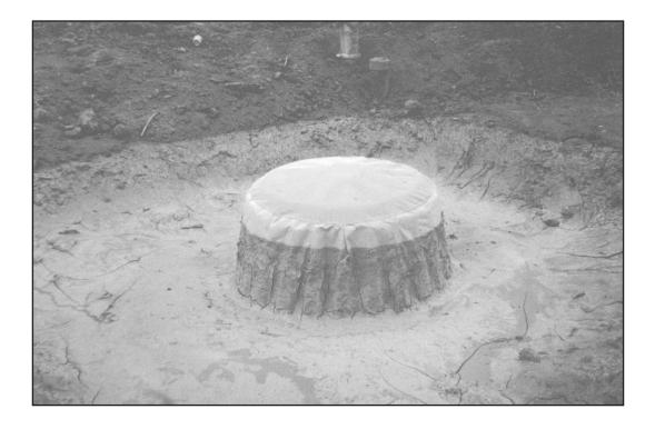
Figure 6-28.7 Equivalent Inlet Sediment Trap
