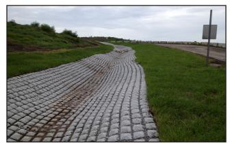
Figure 2.9- This vegetated waterway will safely convey storm water away.
