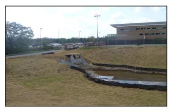
Figure 2.11 - This temporary sediment basin effectively trapped sediment from upstream erosion.
