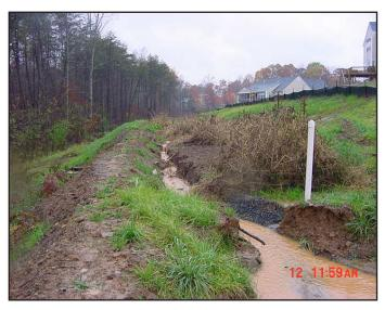
A major issue with conversions is timing. Premature installation of the post-construction practice can result in damage from construction sediments.
