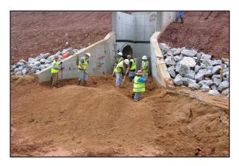
Figure 1.2 - Maintaining outlet protection due to BMP failures higher in the drainage basin.
