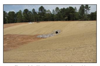
Figure 2.8 - Matting can assist in rapid establishment of vegetation.
