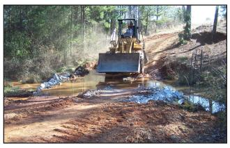
Figure 2.14 - Temporary bridges or culverts should be employed when construction equipment is required to cross natural or constructed channels
