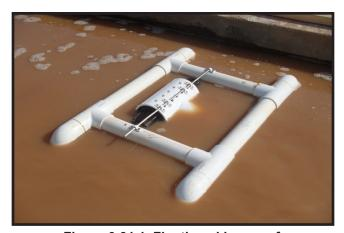
Figure 6-31.1. Floating skimmer of a different design.
