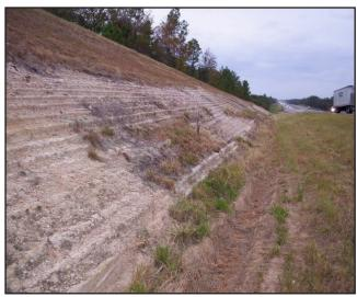
Figure 2.4 - Unstable soil conditions, as on this roadbank, should be avoided.
