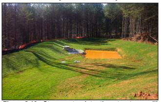
Figure 2.10 - Storm water detention structures will reduce storm water runoff from developed areas.
