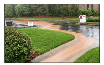
Figure 2.13 - Offsite impact from a neighboring construction site.
