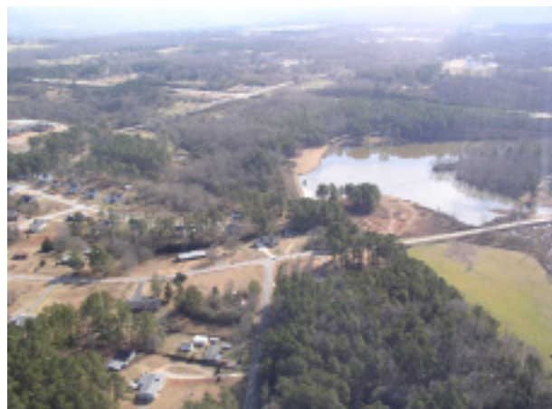
Rehabilitation of the Marbury Creek-22 dam will prevent flooding.
